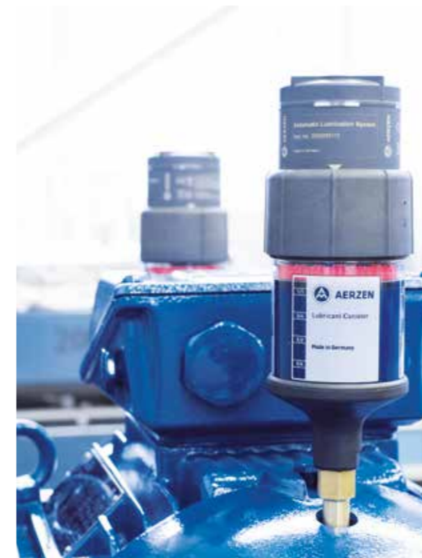
Reduce your maintenance costs – re-lubrication devices from AERZEN
