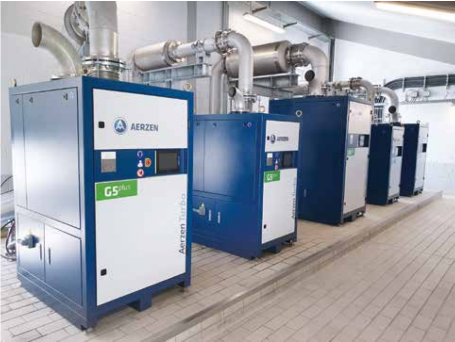
Five turbo blowers from AERZEN ensure the oxygen supply in the aeration tanks.
