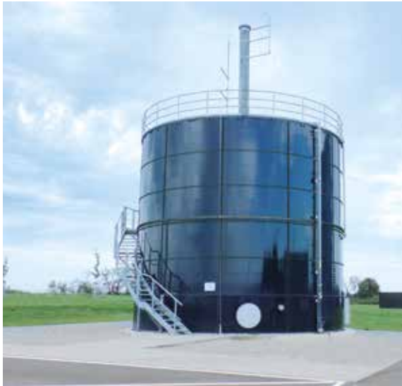
The gas storage tank has a capacity of approx. 500 m 3 .
