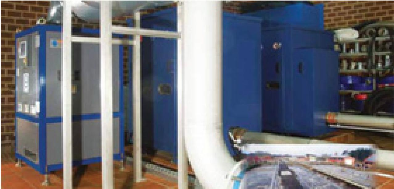
Figure 1 Aerzen AT turbo blower and two PD blowers processing air at a Bremervörde, Germany WWTP.
