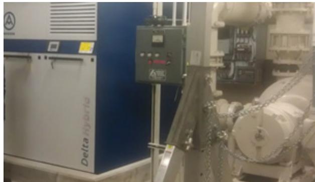
The City of Anacortes replaced a 125HP multistage centrifugal blower (right) with an Aerzen D 62S 75HP hybrid blower (left).
