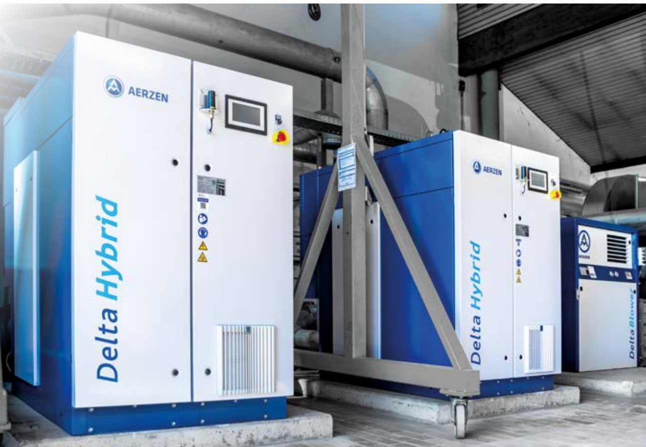
Two AERZEN Delta Hybrid D 31 S screw blowers with direct drive ensure the oxygen supply in the aeration tanks. A Delta Blower GM 25 S positive displacement blower serves as a redundancy machine.
