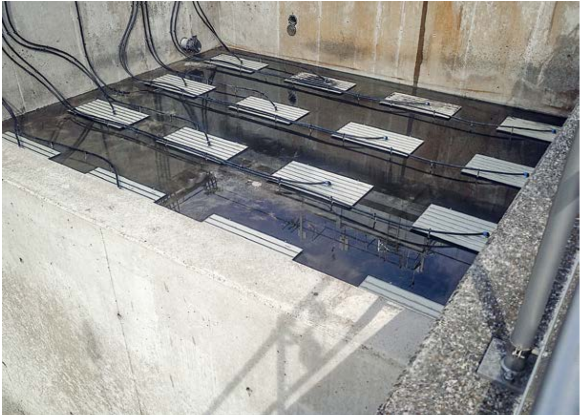
Installation of MESSNER aeration panels®
