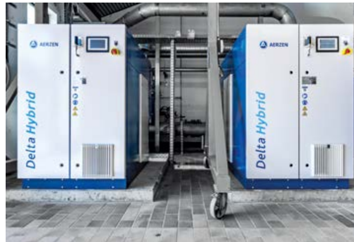
The Delta Hybrid is characterised by very energy-efficient operation and a high turndown. This allows the oxygen supply to be adapted to the load fluctuations of the Unterföhring wastewater treatment plant as required.
