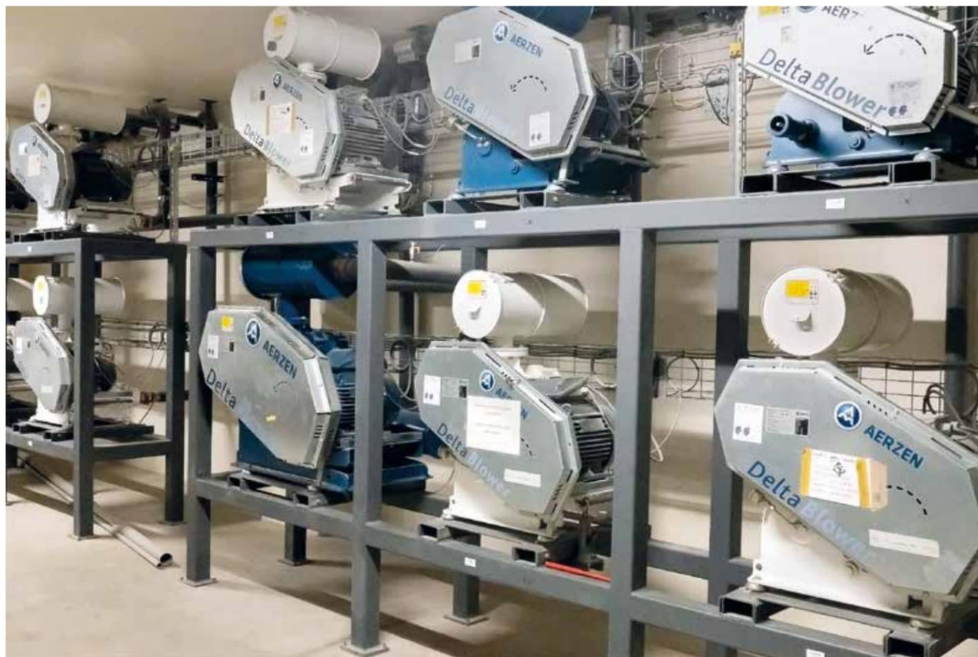
*A total of 21 AERZEN Delta Blower positive displacement blowers keep the flake production going.*
