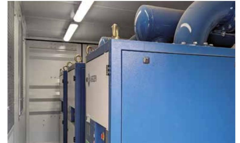
The turbo blowers of the mobile rental solution are state-of-the-art. If required, they can be taken over and permanently installed at the new location of the future wastewater treatment plant.
