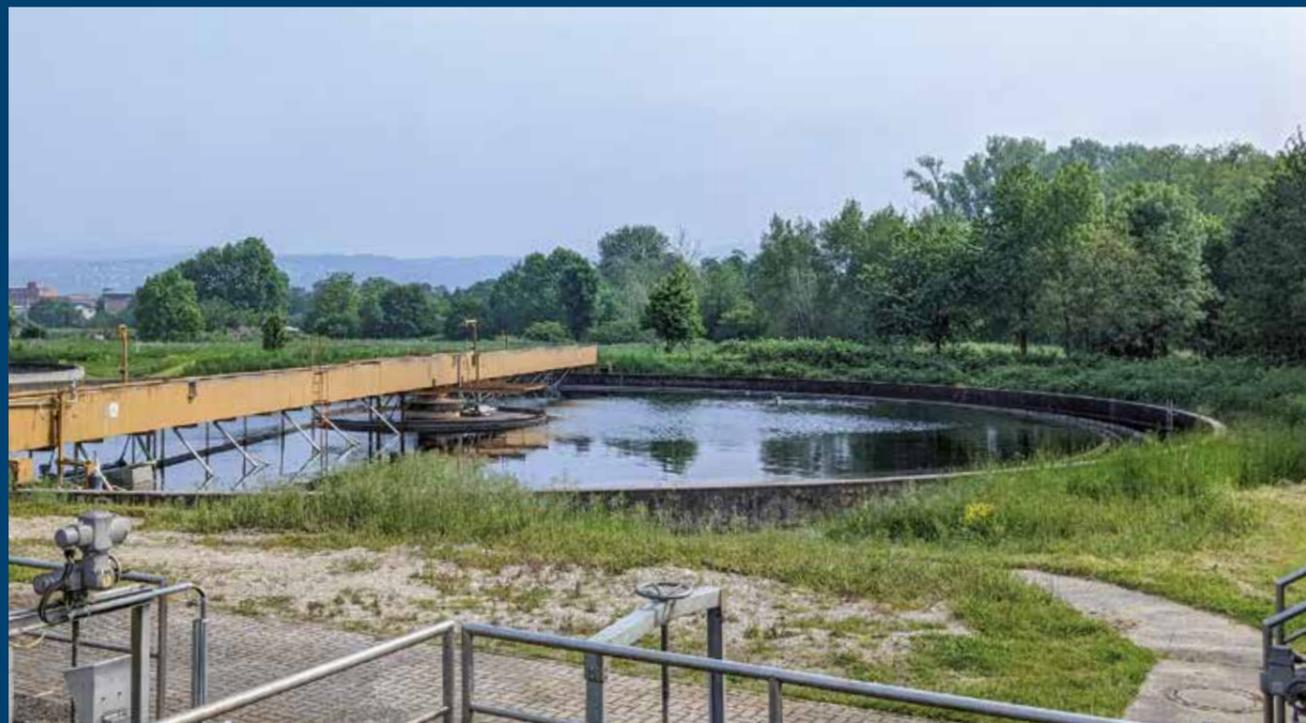
The aeration phase is followed by secondary treatment in the Sinzig wastewater treatment plant in two circular basins.
