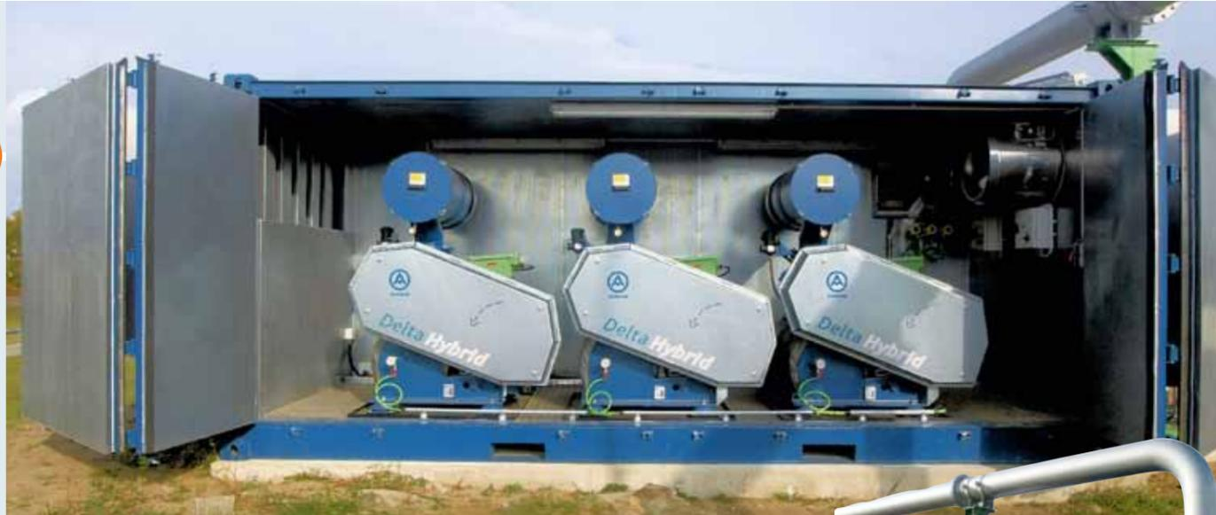
The open doors on the long side of the oxygen-container provide a view of the three Aerzen Delta Hybrid machines.
