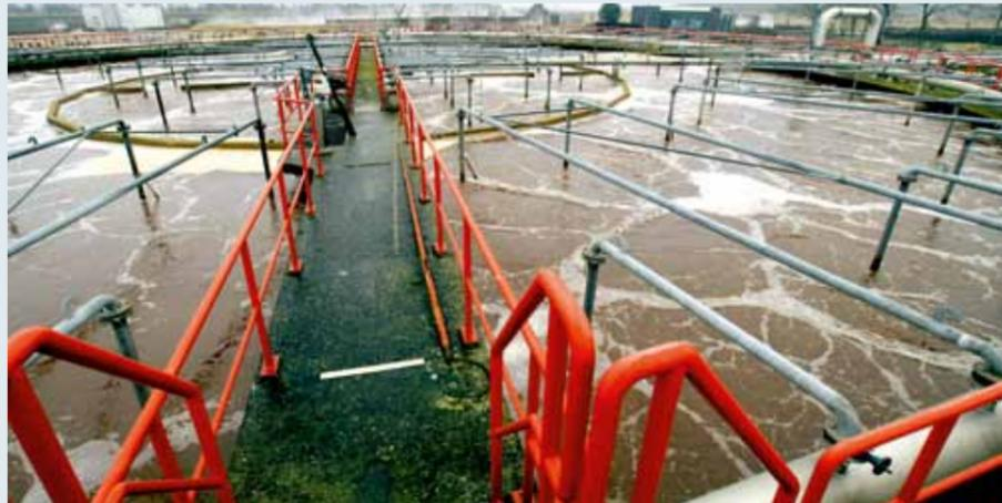
As soon as the oxygen content drops below a set-point value process air is generated.
