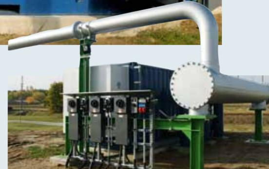
Each rotary lobe compressor can be switched on and off individually from the outside via emergency off switches at the head of the container.
