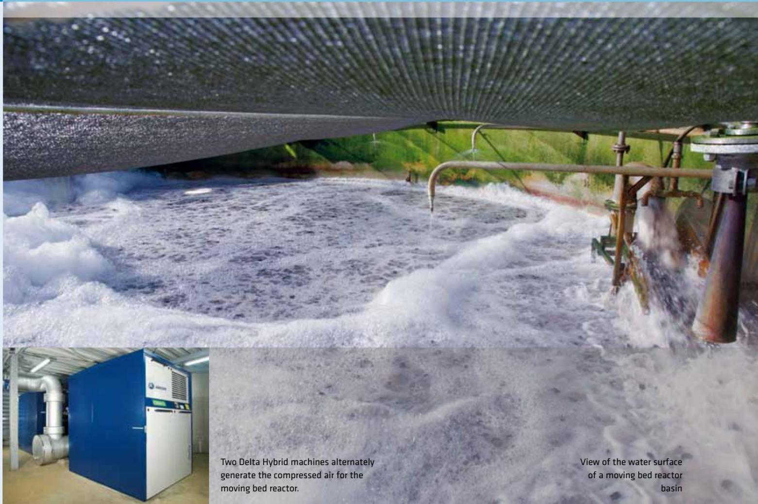
Two Delta Hybrid machines alternately generate the compressed air for the moving bed reactor.
