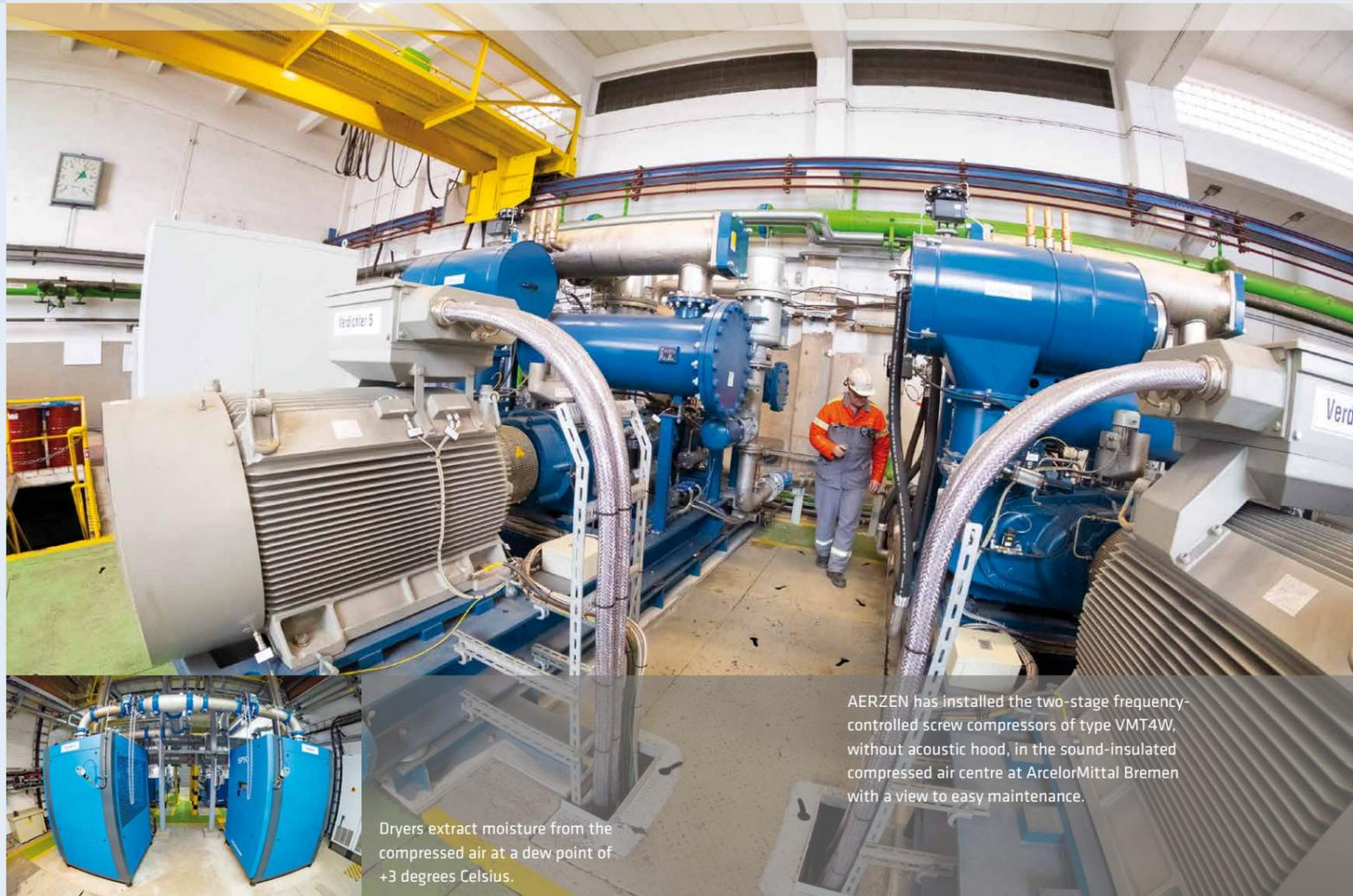
AERZEN has installed the two-stage frequency-controlled screw compressors of type VMT4W, without acoustic hood, in the sound-insulated compressed air centre at ArcelorMittal Bremen with a view to easy maintenance.
