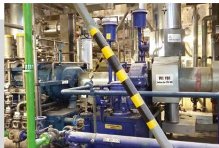
VKO 725S for the compression of lime kiln gas with turbine drive - year of construction 1976.
