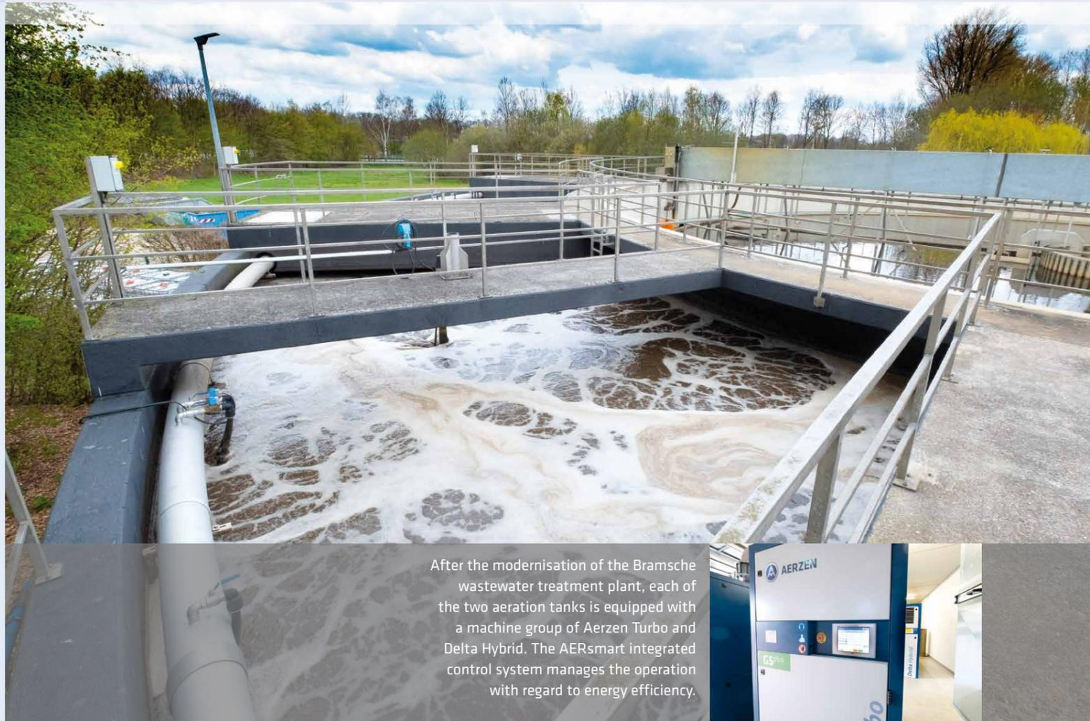
After the modernisation of the Bramsche wastewater treatment plant, each of the two aeration tanks is equipped with a machine group of Aerzen Turbo and Delta Hybrid. The AERsmart integrated control system manages the operation with regard to energy efficiency.
