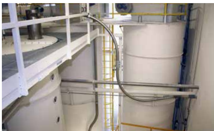
Via the bent silver pipe, the end product enters the pre-silo for bagging.
