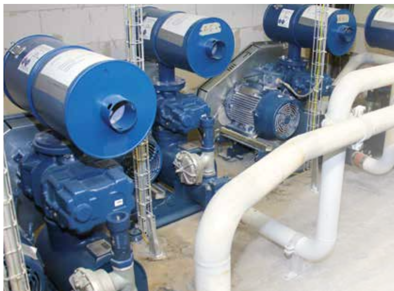
The blower cellar houses the majority of the AERZEN packages.
