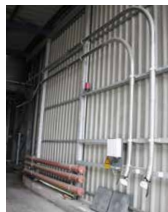
Truck unloading station: AERZEN air is blown into the silo vehicle via one pipe, and the delivered goods are transported into the silos via a second pipe.
