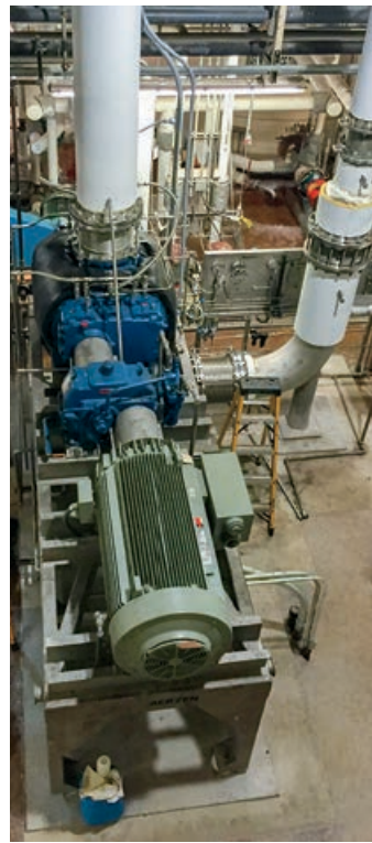
GM 240 S for steam in a ZLD Crystallizer at a battery manufacturer
