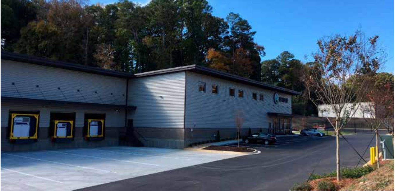
Aerzen Rental machines lined up on the loading dock ready for deployment.
